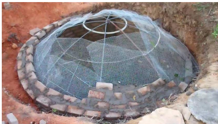
Figure 43: Fixed Dome biogas digester, built by Jacob Chikuhwa
