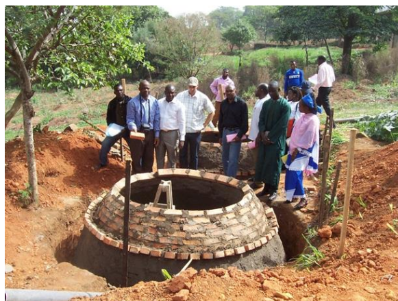
Figure 42: Biogas digester construction (Julius, 2017)
