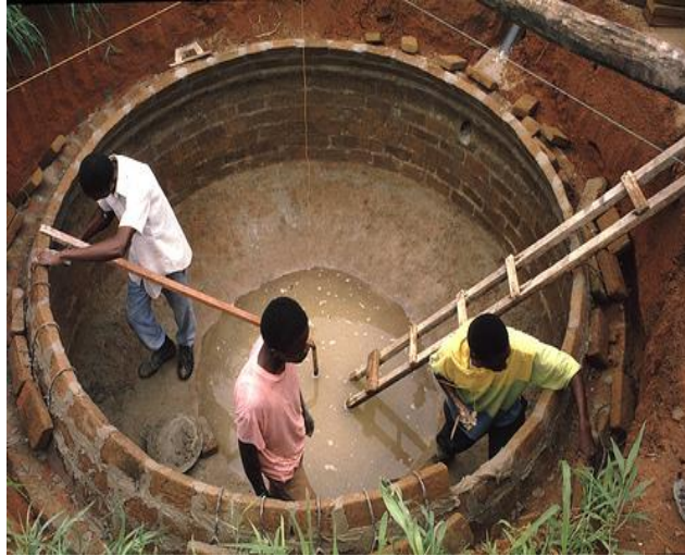
Figure 41: Anaerobic Digester construction (Wilkie, 2015)
